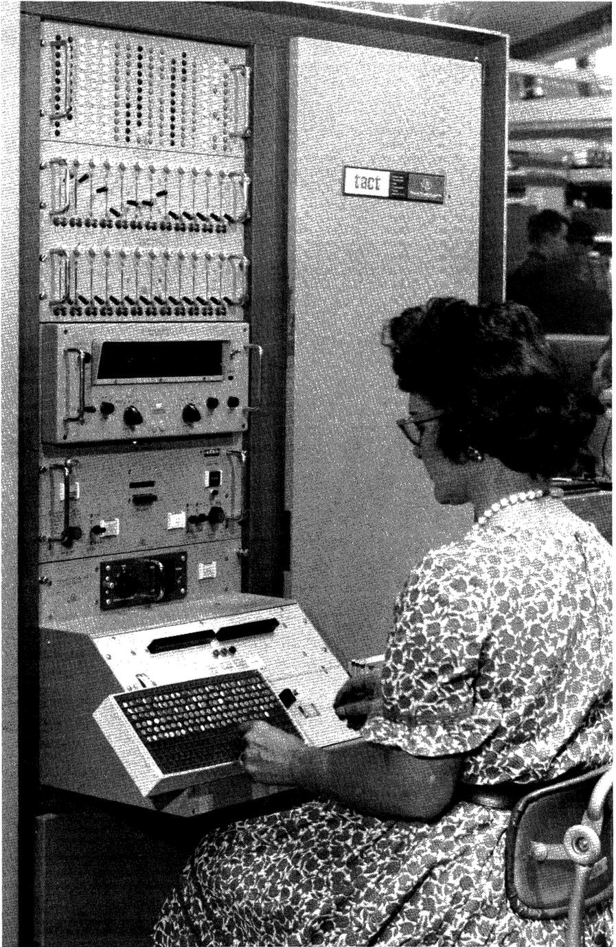
This "TACT," for Transistor and Component Tester, is one of many such TI-designed and TI-built units capable of testing 20 parameters at 7,200 devices per hour.
