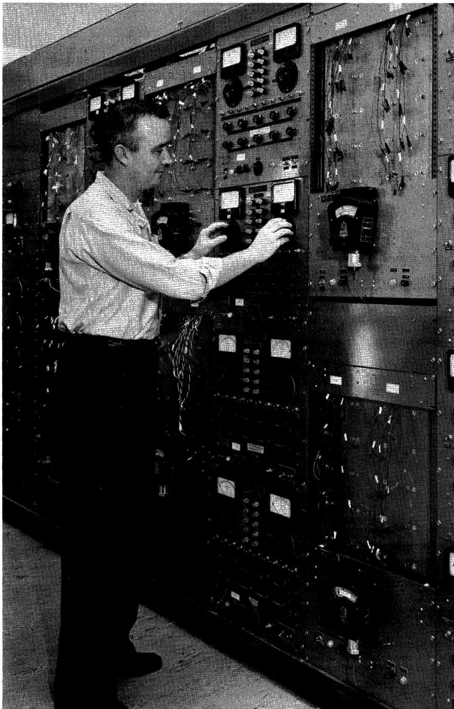
**One small corner of TI's life-testing facilities, where more than 100,000 transistors can simultaneously be subjected to operating life tests.**
