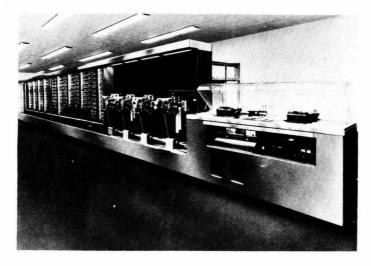
a. Relay Machine: The Harvard-IBM Mark I (Courtesy IBM Corporation)
