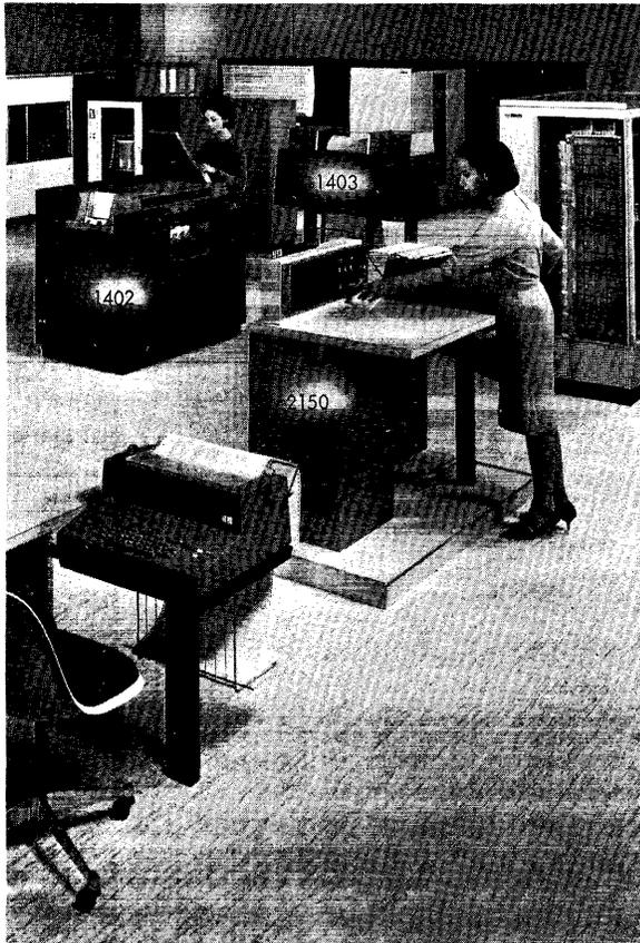
Figure 11. IBM 2150 Console, 1402 Card Read Punch, and 1403 Printer
