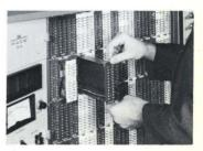
Plug the desired component into the empty position. No re-wiring is necessary.
