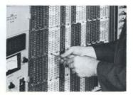
At the front of the computer and with the pre-patch panel removed loosen the two retaining fasteners which secure the component to be replaced.
