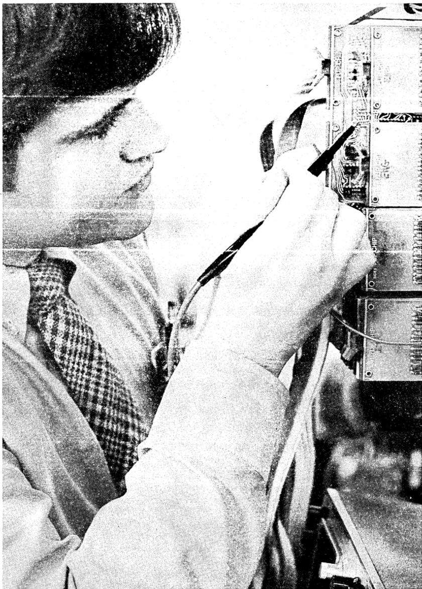
DEC's PDP-14 is designed to be more reliable, more flexible and, in most cases, less expensive than any other electrical system now available for control of machines and systems utilizing two state devices such as limit switches, pushbuttons, motor contactors and solenoids.
