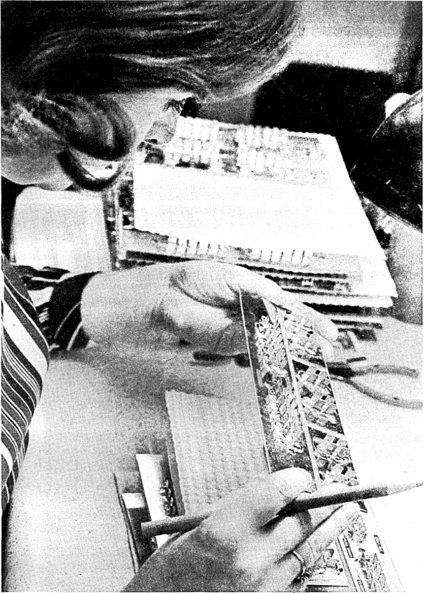
After the modules are flow-soldered, they undergo a visual inspection to insure that all solder points and runs are properly made. If needed, additional solder is added.
