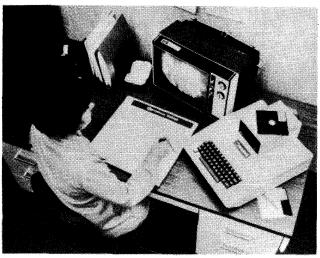
The Apple II configured for fairly typical home use, with single diskette drive and TV set for color graphics monitor. Not as commonly used is the graphics tablet shown here, capable of producing highresolution, multi-colored drawings.
