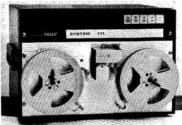
*The Tally System 111 transmits data from punched tape at 120 characters per second and includes reel handling facilities.*
