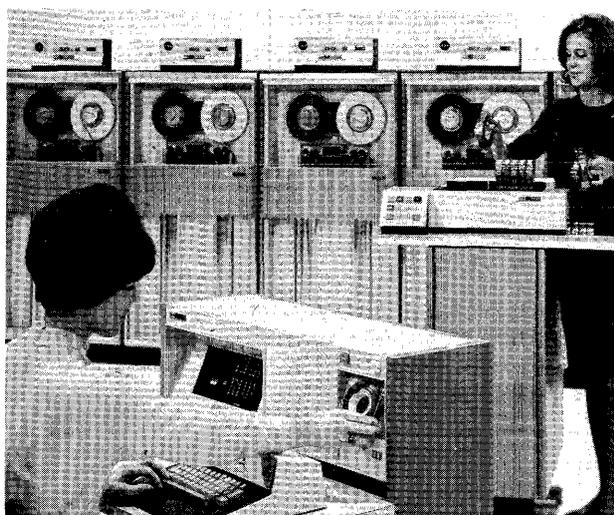
The IBM 2495 Tape Cartridge Reader (right) reads data directly into a System/360 or System/370 computer from cartridges prepared on the Model 50 Magnetic Data Inscrber (foreground).
