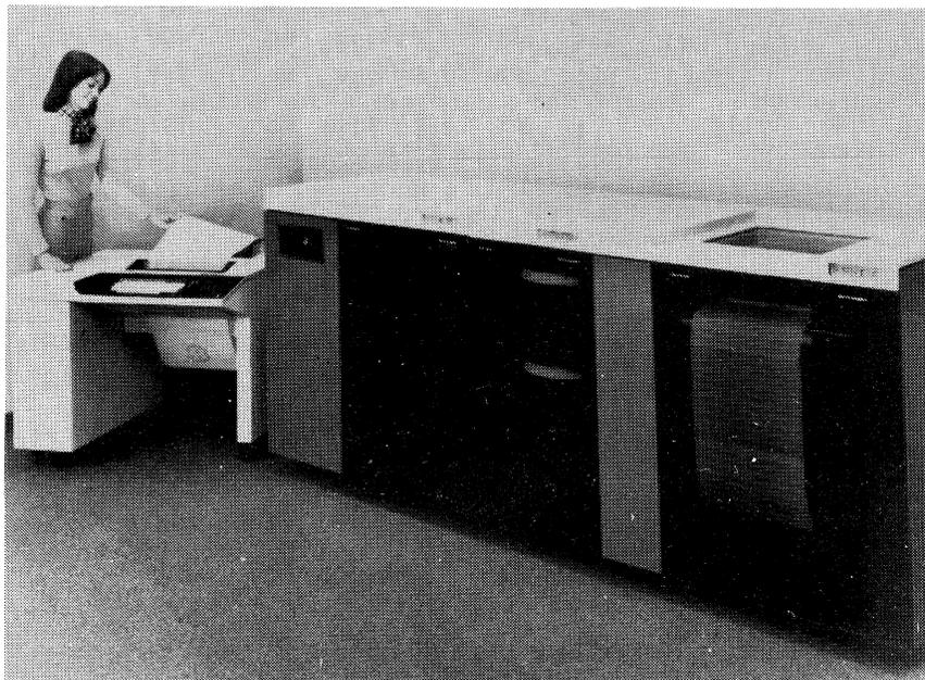
*The B 776 is intended for larger Burroughs computer systems. Using a different internal architecture than the B 774, it can also handle up to 32 lines and, in addition, has capabilities for including local peripheral devices, as shown above, and user programming.*
