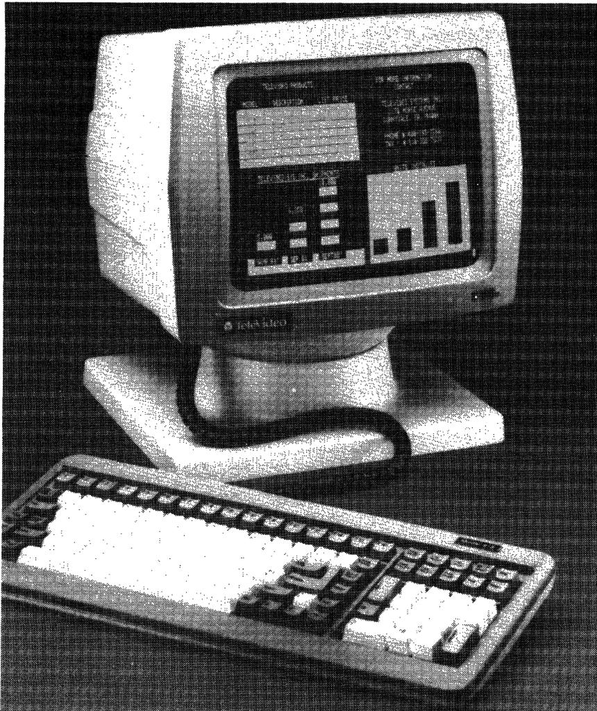
*TeleVideo has introduced a new display terminal enclosure design which features a tilt/swivel screen, reduced footprint size, and a low-profile detached keyboard. This design is implemented on three new models, the 914, 924, and the soon-to-be-available 960.*
