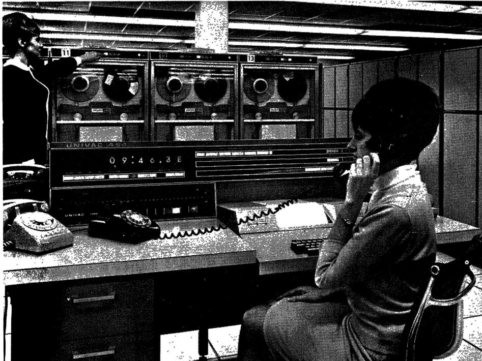
Figure 1. Control Console of the UNIVAC 494 Real-Time System.
