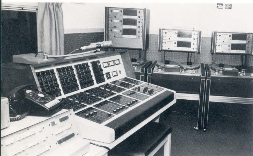
Interior of the recording control room of The United States Army Band at Ft. Myer, Virginia, showing a bank of master recorders in the background. The main console is a twelve-position, three-channel custom unit.
