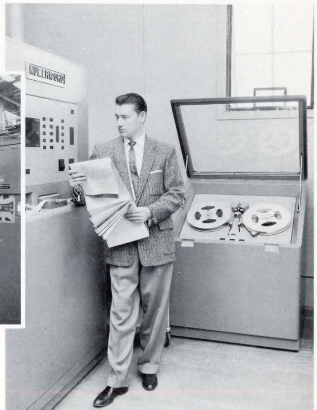
A Giddings & Lewis numerical profiler for manufacturing components for the F-102A supersonic interceptor at CONVAIR, San Diego. Inset shows director facility for converting information from punched-paper tape to magnetic tape, which then controls operation of the automatic profiler.
