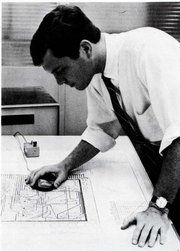
**Automation** in the manufacture of PC boards has advanced to the point where not only the artwork, but even the tooling, can be determined and controlled by the computer. Here a layout is digitized to feed the inputs to the computer (Photo courtesy of Photocircuits Corp.).
