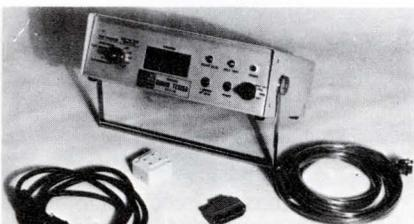
This pre-set, bit-count modem tester determines error rates on asynchronous modems to 240 hps and synchronous modems to 200,000 bps. Designed for both local and remote looped, full duplex modems, it is compatible with all RS232B interfaced modems. Sanders Associates, Inc., Daniel Webster Hwy, So., Nashua, N.H. 03060. (603) 885-2816.
