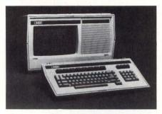
nations. The keyboard can be detached from the terminal or folded and locked for security and portability. The model 831 offers asynchronous point-to-point communication in full and half duplex, with separate keyboard-selectable transmit and receive rates from 50 to 19.2K baud. The terminal can be upgraded to a CP/M-based 8-bit microcomputer. Price is \$1395 in single-unit quantities, with volume discounts available. Direct Inc.. 4201 Burton Dr., Santa Clara, Calif. 95050. Circle No 326
