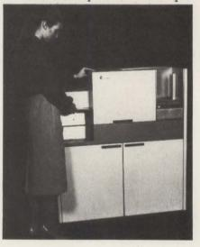
hopper and output stacker have a capacity of 1000 cards each. Card-punch verification is accomplished through echo-check error detection. A 100-card-capacity reject stacker automatically selects cards that do not pass the echo-check verification. Control software is compatible with Data General operating systems. The punch also includes an interface cable and controller board that plugs directly into the backplane of the DG Nova. Price is \$12,500, with
