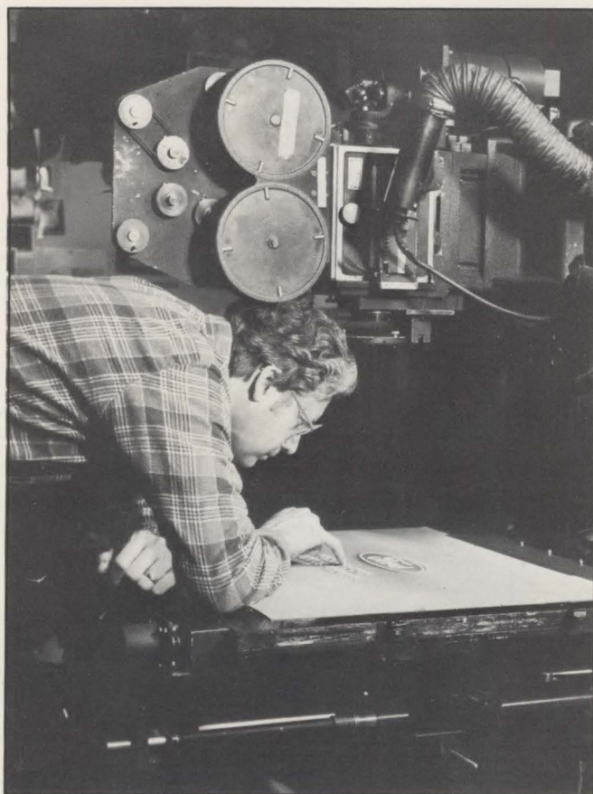
Once a matte or title has been correctly positioned on the animation stand, the Cinetron system aids in computer animation. At CFA, the time required for a zoom-in on a piece of artwork requiring 10 ft. of film has been cut from 3 hr. to 20 min.
