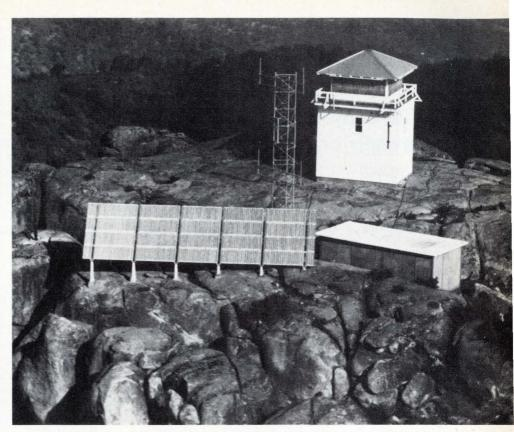
**5. The size of things to come?** Powering a communications link on a mountaintop in southern California is a solar-energy conversion array from Spectrolab. Approximately 900 square feet in area, the array produces well over 3 kilowatts of peak power. A big advantage of this kind of power source is that it can be left unattended.
