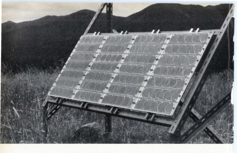
meters of water and is popular because it does not drain the water table too quickly. A high-power thermal pumping unit drains the well after a few minutes in the desert regions near Algeria and Tunisia, where the water table is 20-30 meters deep. The photovoltaic-powered pump provides a slower, steadier flow, has low maintenance, and costs about the same.
