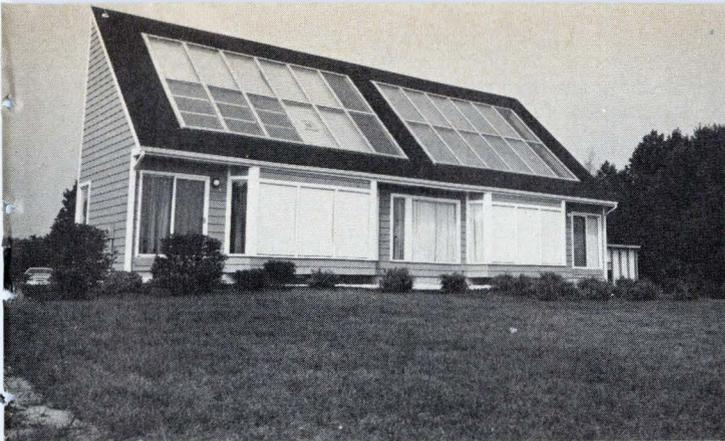
**6. Test house.** Under direction of Karl W. Böer (right), Institute of Energy Conversion has built Solar One, an experimental house for testing solar-heating and cooling methods and cadmium-sulfide solar cells (the darker panels at lower left on the roof).
