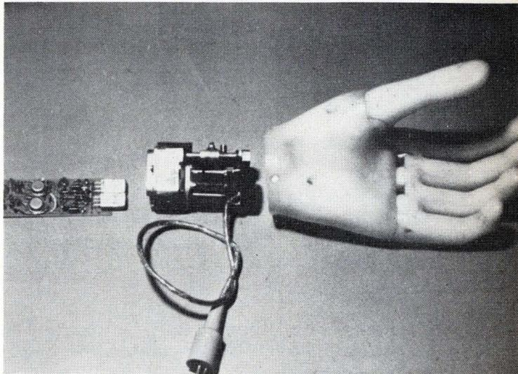
**Improvement.** Closeup of prosthetic hand and drive motor with IC control unit. Design successfully overcame shortcomings of Russian prosthetic hand, which suffered frequent breakdowns because of poor-quality components.
