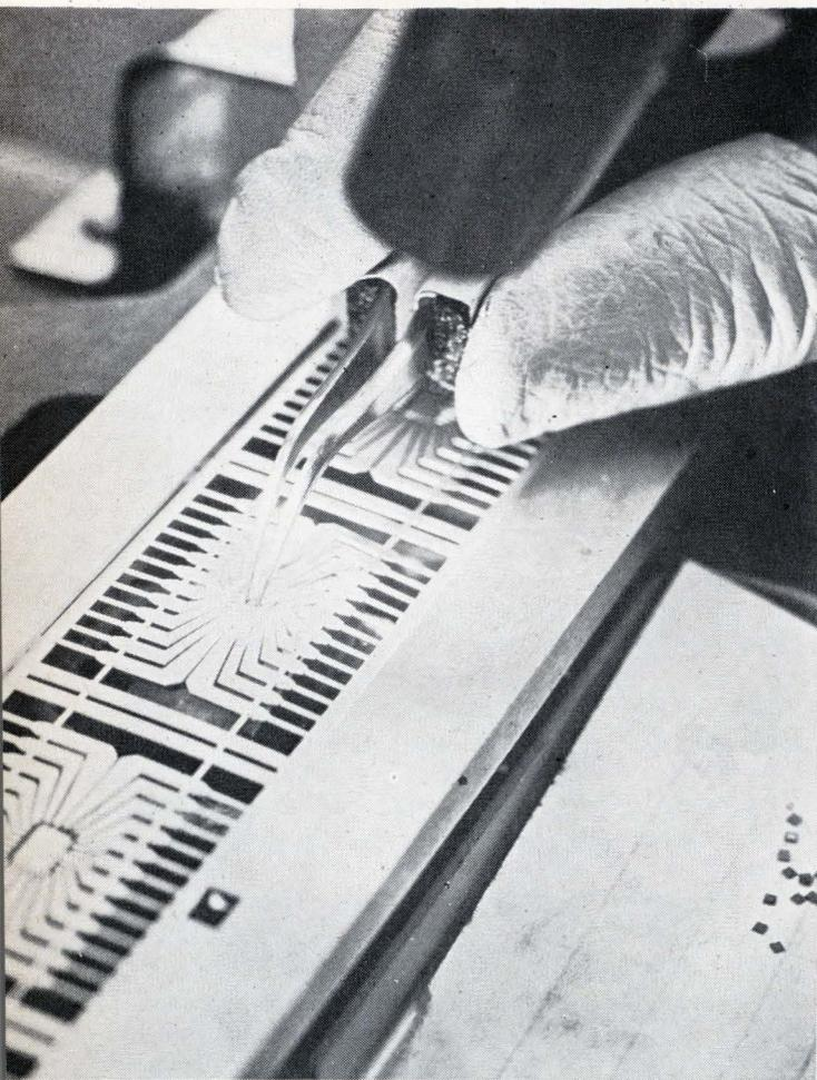
**Cost-squeezing.** Packaging of linear IC's into low-cost, nonhermetic-sealed, dual-in-line packages (DIP) is a primary means of bringing device costs down. At TI's Dallas facilities four of every 10 IC's made this year will be plastic-encapsulated types. The same monolithic chip used in metal cans and flatpacks (such as this SN52709 amplifier) is placed onto DIP carriers; subsequently, each molded package is cut into a separate unit.
