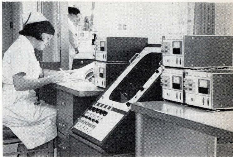
**Central monitoring station.** Five-bed cardiac care unit is watched over by one nurse. Multichannel scope simultaneously displays each patient's EKG. Individual units display patient's heart rate on a meter, and lighted indicators warn of significant changes.
