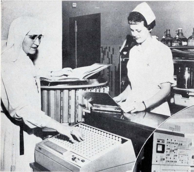
**Data inputs.** Terminals like this will permit personnel at hospital stations to transmit data on patients' functions, such as pulse rate, blood pressure, and temperature, to the central computer.
