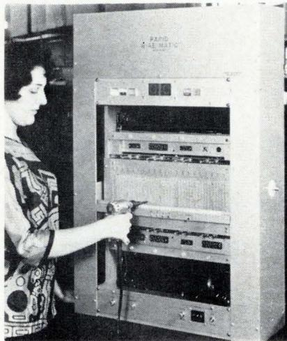
**"It makes sure** the wiring is right the first time," says company president Saul Liss describing a system that automatically guides the routing and terminations of wires in a back panel or harness, and tests the connections as they are made. "The system is designed to eliminate inspection, debugging and reworking of what should be a finished product," he asserts.
