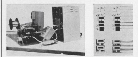
Lead material is fed from spool at left to carriage and welding head. At right are typical microcircuits with soldered leads.
