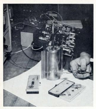
**Components** for a radiation-hardened missile-borne amplifier undergo extensive testing at General Electric Co.'s Reentry Systems division. Metal cannister contains amplifier modules shown on the cover.
