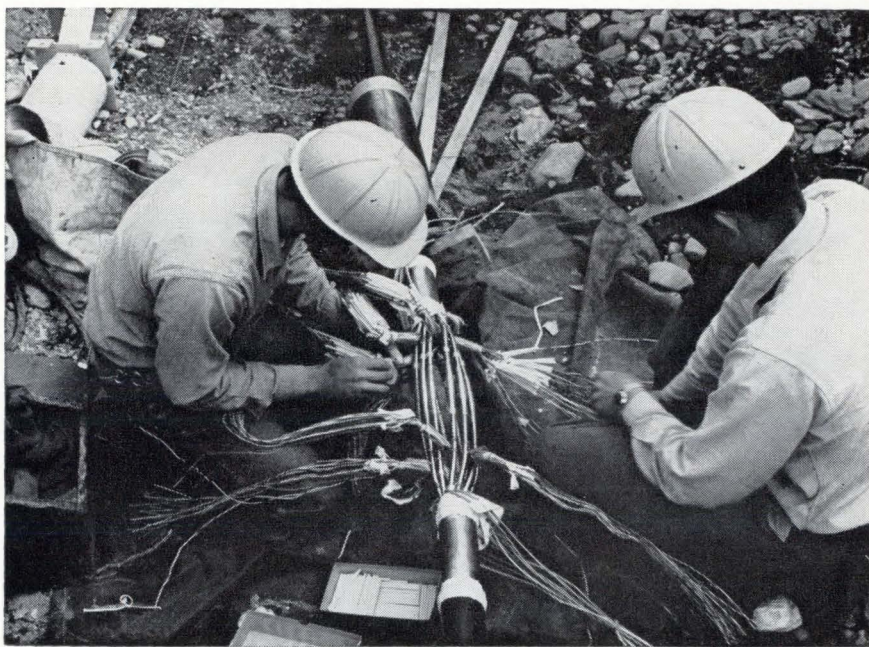
Two sections of Bell System's blast-resistant cable are spliced to join the East and West Coasts. The 12-tube coaxial link provides six sets of 1,860-channel circuits and two spare sets in case of failure. Wires carry alarm and control circuits.
