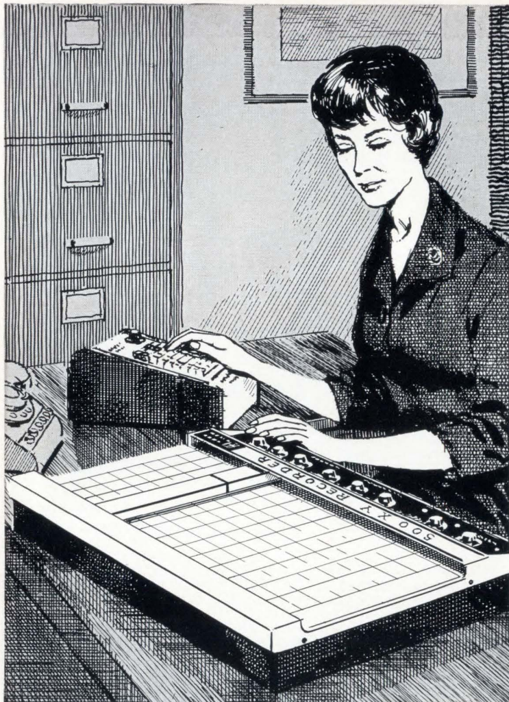
Secretary, using key board and EI X-Y Recorder, now handles engineering laboratory plotting work as part of her typing function.
