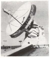
OVERHEAD tracking and communications with Relay satellite will be the specialty of this 40-foot-dish antenna system. It will be the Relay project's western terminus near Barstow, Calif. Built by Philco for NASA, it has a double-elevation mount, does not move in azimuth. Three-channel monopulse receiver, servo and digital equipment are all solid-state
