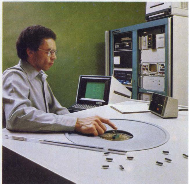
Graphic displays of test results are one benefit of computer-controlled test equipment. Evaluation of LSI circuits is shown here on the Tektronix S-3260.
