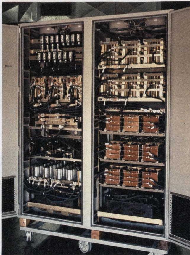
kVA UPS (left). The system includes a rectifier/charger, inverter and static and manual switches (right).
