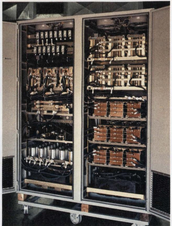
kVA UPS (left). The system includes a rectifier/charger, inverter and static and manual switches (right).
