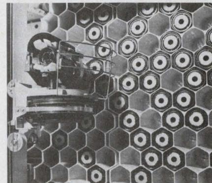
Vast amounts of data can be stored on data cartridges housed in the honeycomb storage compartments of the IBM 3850 mass storage system. Two cartridges can store the same amount of data as one disc pack.
