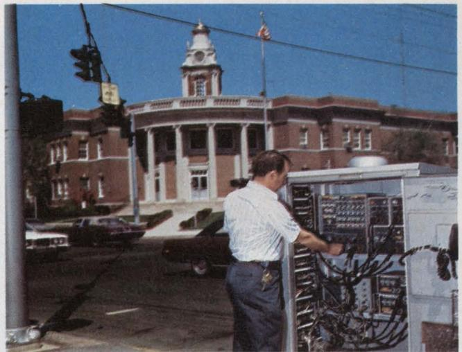
This traffic controller is a key element in a Connecticut system by Automatic Signal, Norwalk, that cut travel time by 45% through a high-traffic shopping district. Local intersection control is exercised by a CMOS microcomputer that talks to the system computer.
