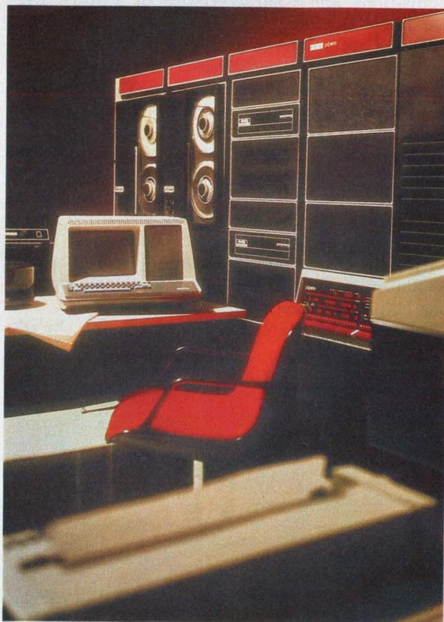
Digital Equipment Corporation's new midcomputer, the PDP 11/70, employs a special memory architecture in which a 2 k byte bipolar cache memory acts as a buffer between main memory and the unit's general purpose registers. 32-bit internal data paths carry data to and from the cache memory, permitting data transfers between memory and registers to approach the 300-ns execution time of the central processor.
