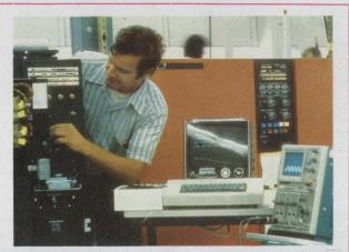
The finished product tests other System/7's at IBM before shipment. The System/7 under test (left) is linked to the computer that monitors memory operation, control functions and data flow. Test data are printed out on a console (right, background) and relayed to a central System/360. A single System/7 can test up to four processors.
