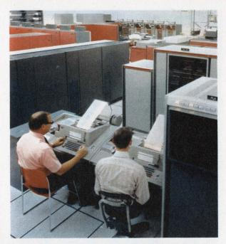
The Collins C-System uses a localized high-speed ring to join hosts and storage devices. Low-speed loops drive terminals and input devices. The system shown provides a statewide lowa police network, with access to more than seven million traffic records and 250,000 criminal records on file in a System/370 complex at Des Moines.
