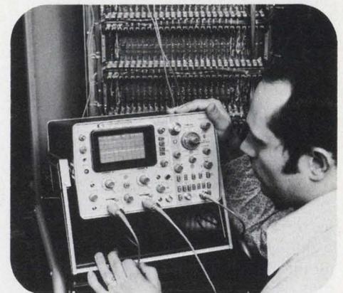
The portable 1703A scope on-site at Utah Power and Light Company.
