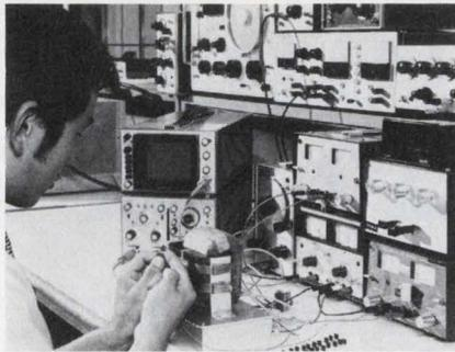
An engineer at Matsushita tests some of the company's new, monolithic Hall-effect ICs.
