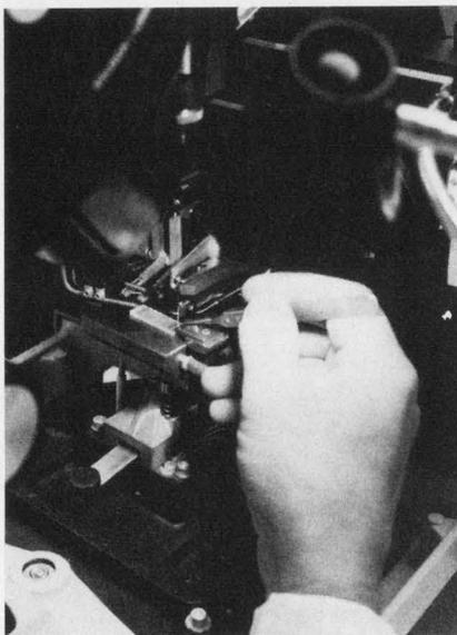
In a special clean room at Fort Monmouth a technician bonds leads to two transducers on a surface-wave dispersive delay line. The device might be used in a radar to determine range resolution.
