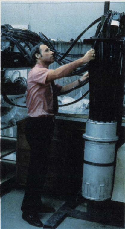
**Electrical penetration conductors at Gulf take data from sensors inside a reactor's core through the containment wall to a display.**
