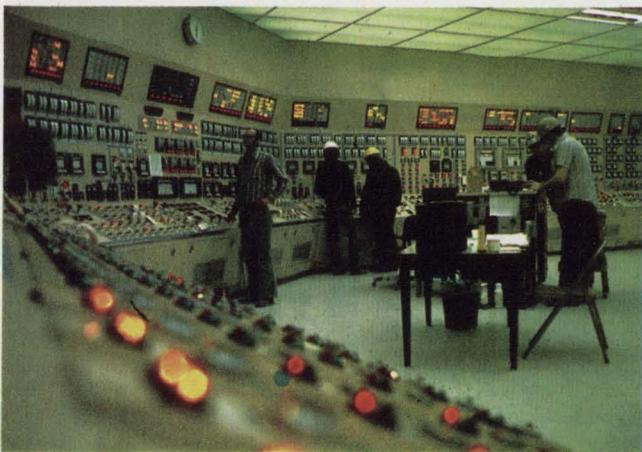
Control room at Commonwealth Edison's Dresden reactor in Morris, Ill., was built by General Electric. It displays data from sensors throughout the plant.
