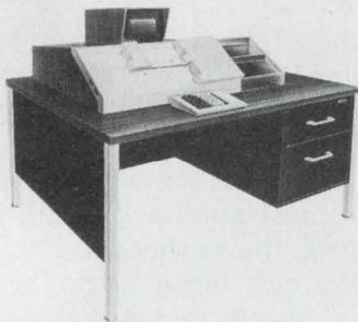
Inforex is using an Intel micro computer in a system that processes incoming bill-paying checks for banks, retail stores, credit card companies and the like. The system reads the return portion of the bill with a numeric optical scanner, endorses the check for deposit and records the entire transaction on magnetic tape. By performing several clerical tasks at one station under the control of one operator, the system speeds processing and greatly reduces clerical costs.
