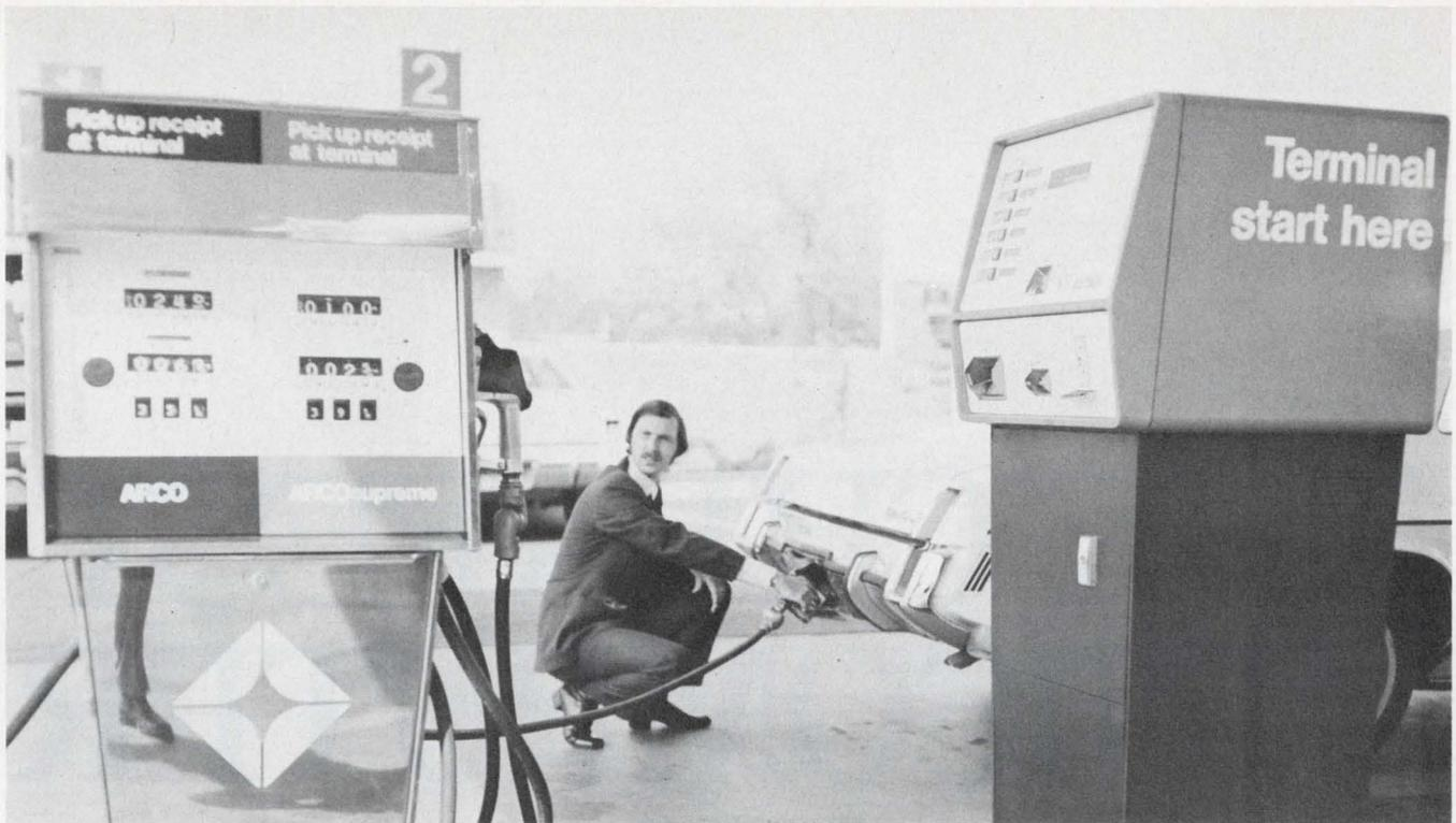
In the world's first computerized self-service gasoline station at Lawndale, Calif., each pump is connected to a terminal that houses a minicomputer (right). The terminal accepts either money or a credit card. A card that is inserted is automatically checked for the customer's credit rating. If his credit is good, he gets to pump
