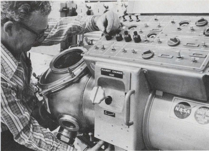
**Manufacturing facility** in Skylab consists of a vacuum work chamber 16 inches in diameter with four-inch-diameter opening to space. Tests will include electron-beam welding, crystal growing and metals melting.
