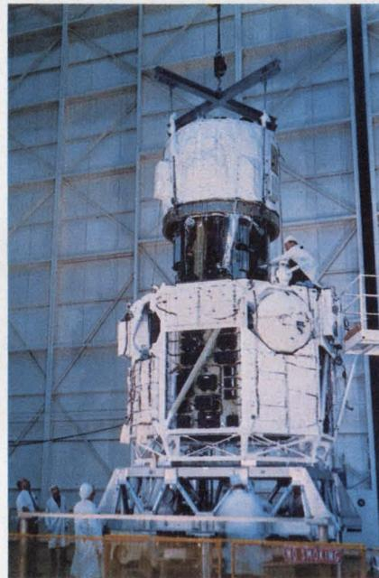
Apollo Telescope Mount canister is being lowered into its outer cluster. The solar observatory weighs 24,650 pounds, contains eight telescopes.
