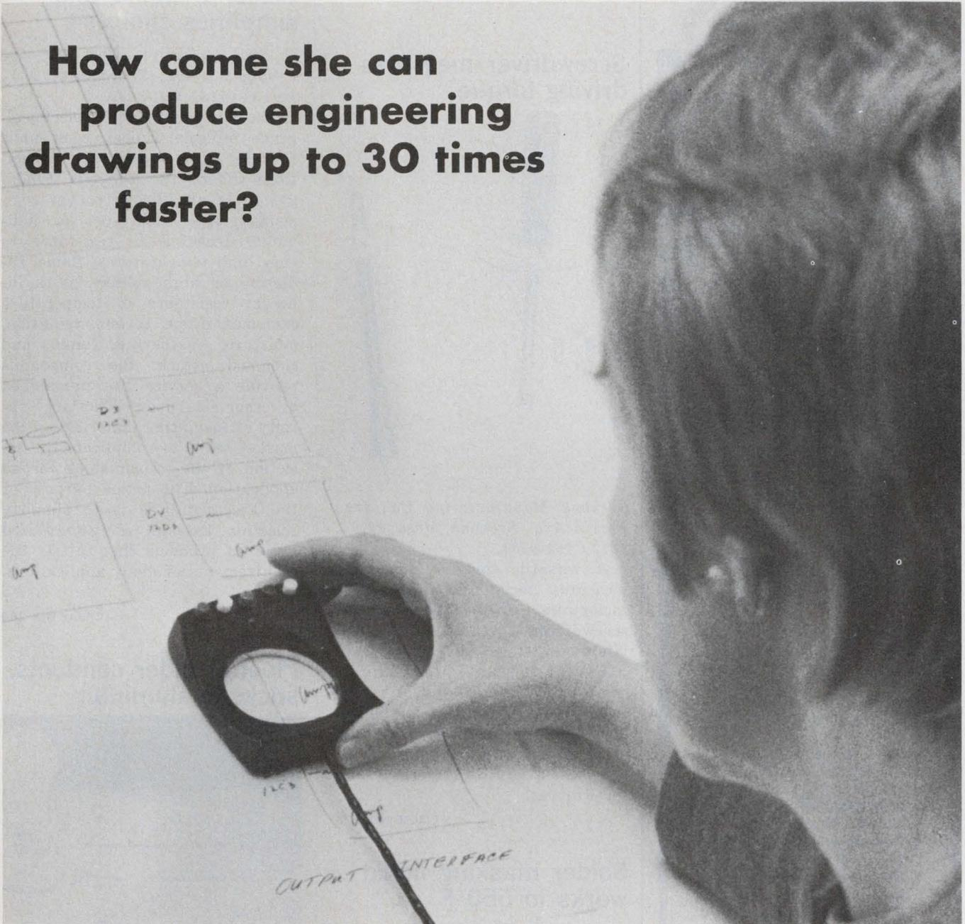
It's simple. She has a Bendix Interactive Drafting System 100. It constructs precise engineering drawings from rough sketches a whopping *five to thirty* times faster than conventional methods.
