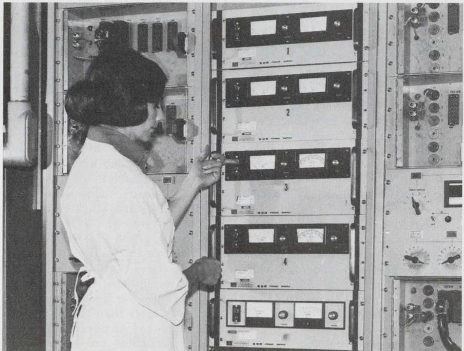
Five of E/M's 5 KW SCR Power Supplies are used in General Electric's electrolytic capacitor aging system.
