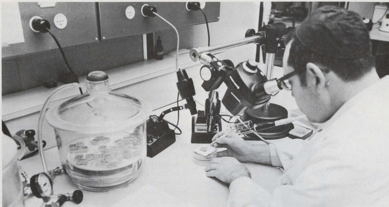
**Technician inspects hybrid thin-film module** produced at Elta Electronics Industries Ltd. in Ashdod. Thin and
