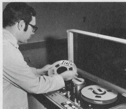
New "High Energy" tape being placed on video helical recorder is treated with a cobalt-modified ferric oxide formulation that creates a 4-dB increase in both rf output and signal-to-noise ratio. The 3M Co. will use the new material on video tapes, sound cassettes, and instrumentation and computer tapes. Above are the oscilloscope readings of rf output of standard tape (left) compared with almost double the output (right) of the tape backed with the new oxide.
