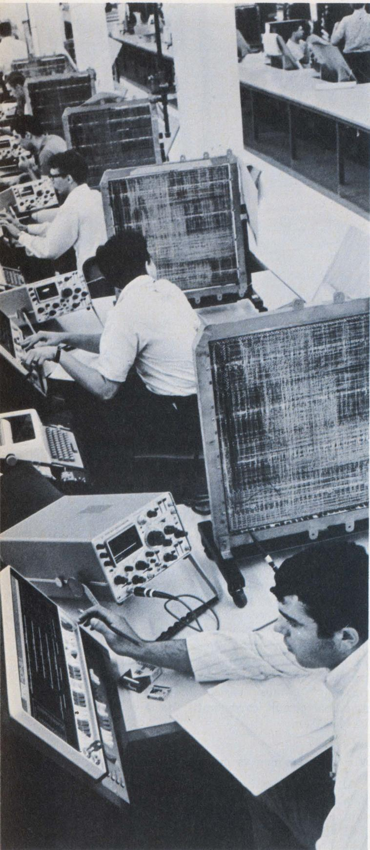
**Minicomputers** are used to test minicomputer subassemblies at the Digital Equipment Corp., Maynard, Mass. Besides performing all the tests, a hard copy of the results becomes part of the documentation of each part. The Digital plant now probably has the highest concentration of test minicomputers everywhere.
