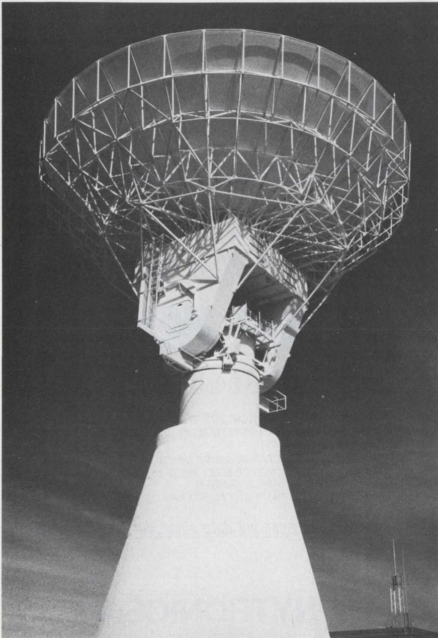
Rampart S-band radar acquires reentering payload, measures cross section and trajectory, then passes directional data on to RAM radar.
