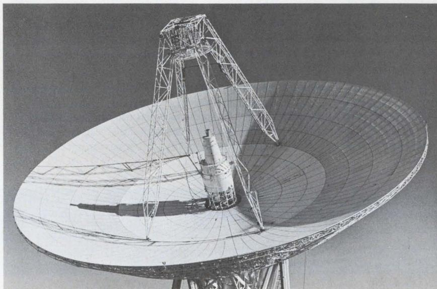
Transmission of data from Mars at 16,000 bits per second became feasible when a 210-foot antenna went into operation. The result: best photos yet taken of the planet. p. 25.
