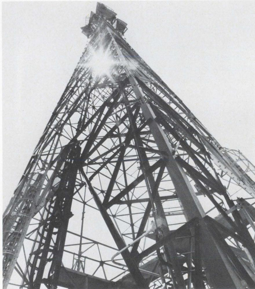
Radio relay tower for Bell's TH3 microwave system. TH3 transmits 10,800 simultaneous telephone conversations.
