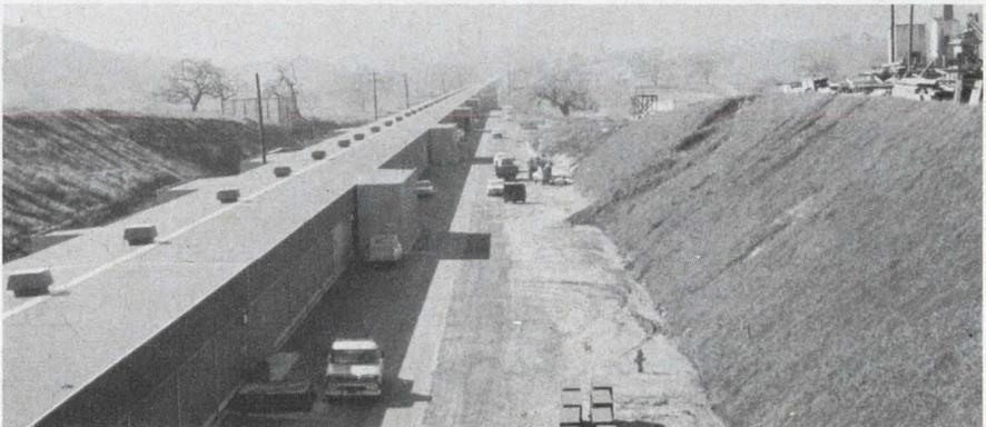
**SLAC comprises two main elements**, both extending over the 2-mile length. The accelerator housing (left) is an 11-foot-wide by 10-foot-high underground tunnel that contains the accelerator proper and related systems. The klystron gallery (right) is a 29-foot-wide by 13-foot-high above-ground installation containing the klystrons, modulators, vacuum pumps and other auxiliary equipment.
