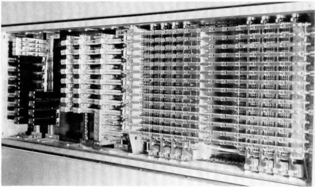
Figure 13 - Pentaconta terminal selector frame for 104 subscriber lines.
