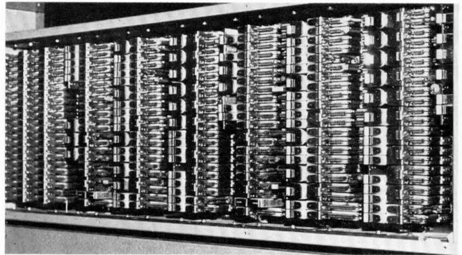
Figure 12 - Pentaconta marker frame with 2 markers.
