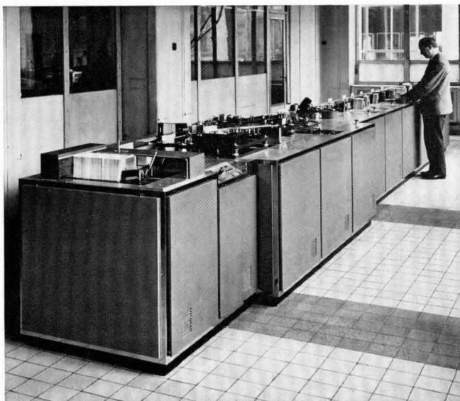
Automatic indexing machine used for presorting envelopes in postal cheque office.
