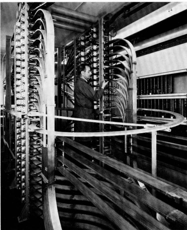
Switching facilities for pneumatic tube distributing system that handles toll tickets without carriers.
