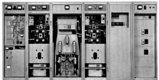
Figure 1 - Design of the 10,2-kilowatt television transmitter (from left to right): vision/sound driver stage, klystron vision amplifier, combining unit, klystron sound amplifier, high-voltage unit, and cable distribution rack.
