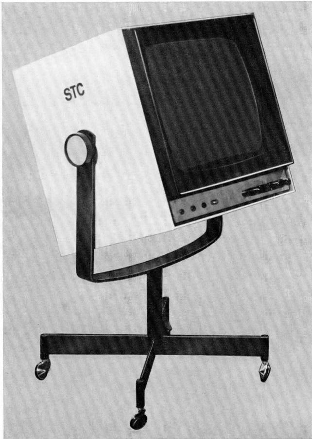
The castor-mounted cradle floor stand enables this 19-inch closed-circuit-television monitor to be given almost any orientation.
