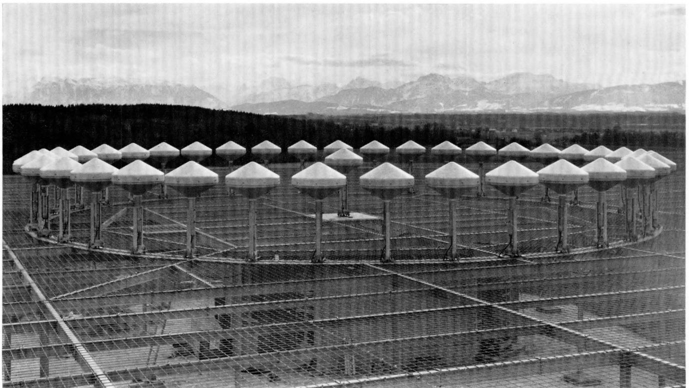
Figure 9 - Doppler very-high-frequency omnidirectional range antenna at the ground station near Salzburg, Austria.
