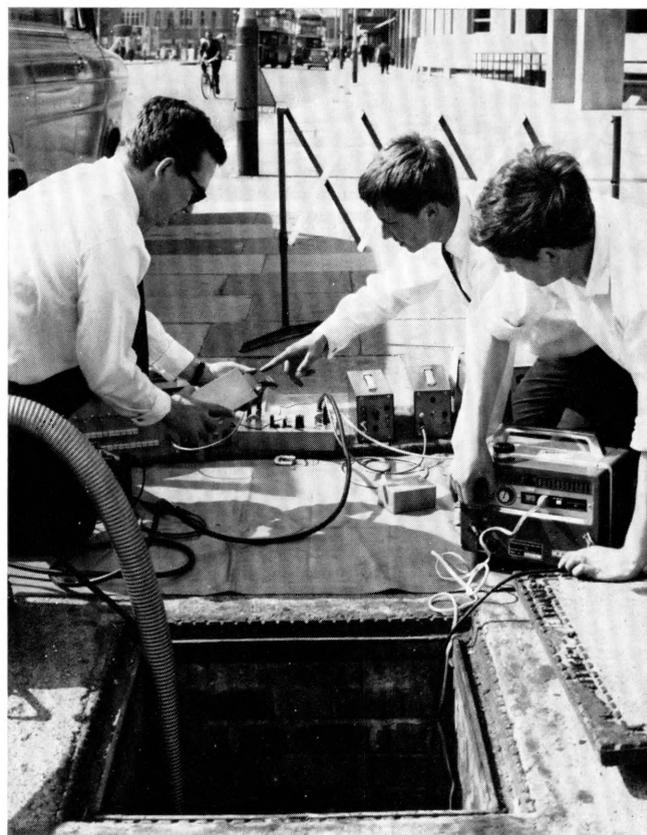
Engineers from STC's Installation and Maintenance Service Division, Balsdon, at work on the first PCM installation in London's Waterloo Road.
