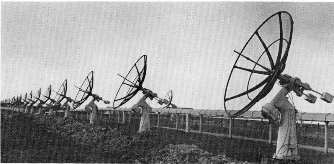
Figure 15—View of some of the 48 antennas making up an interferometer system for solar and galactic radioastronomy.
