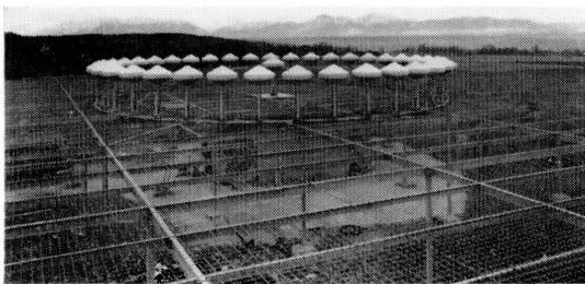
Figure 16—Circular array of 39 radiators for the Doppler very-high-frequency omnidirectional radio range near Salzburg, Austria.
