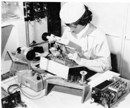
Figure 2—Operator assembling conventional components to a printed-circuit board, which already has flat packs welded on to the opposite side. A complete *STR 70-P* unit with covers removed is in the lower right corner.
