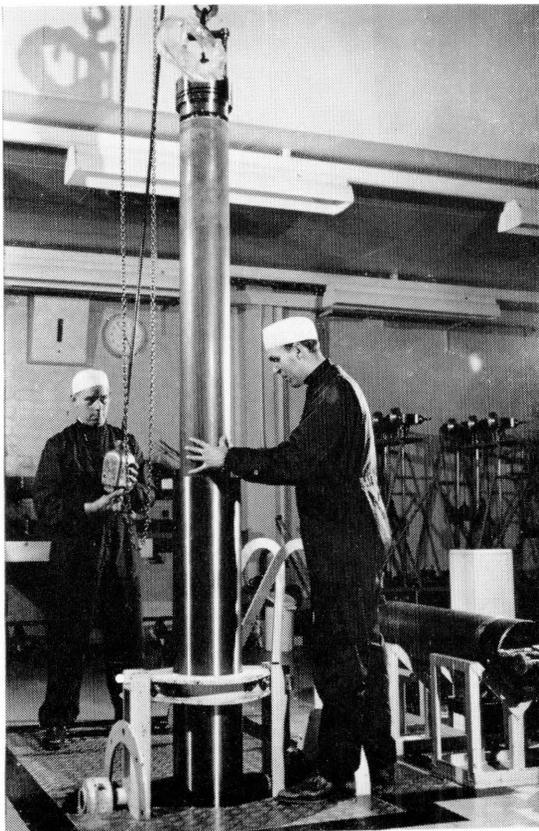
Figure 5—Telephone repeater capsule being lowered into the high-strength steel case that can withstand sea-bottom pressure preparatory to undergoing testing before being accepted for service.
