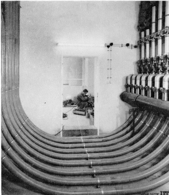
Figure 9—Receiving pneumatic tubes at Schiphol Airport.
