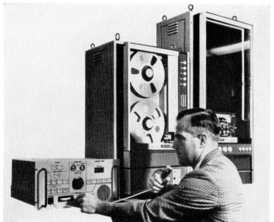
Figure 12—Sonar data recorders. The two tall cabinets house magnetic tape recorders and the smaller cabinet holds the control equipment.
