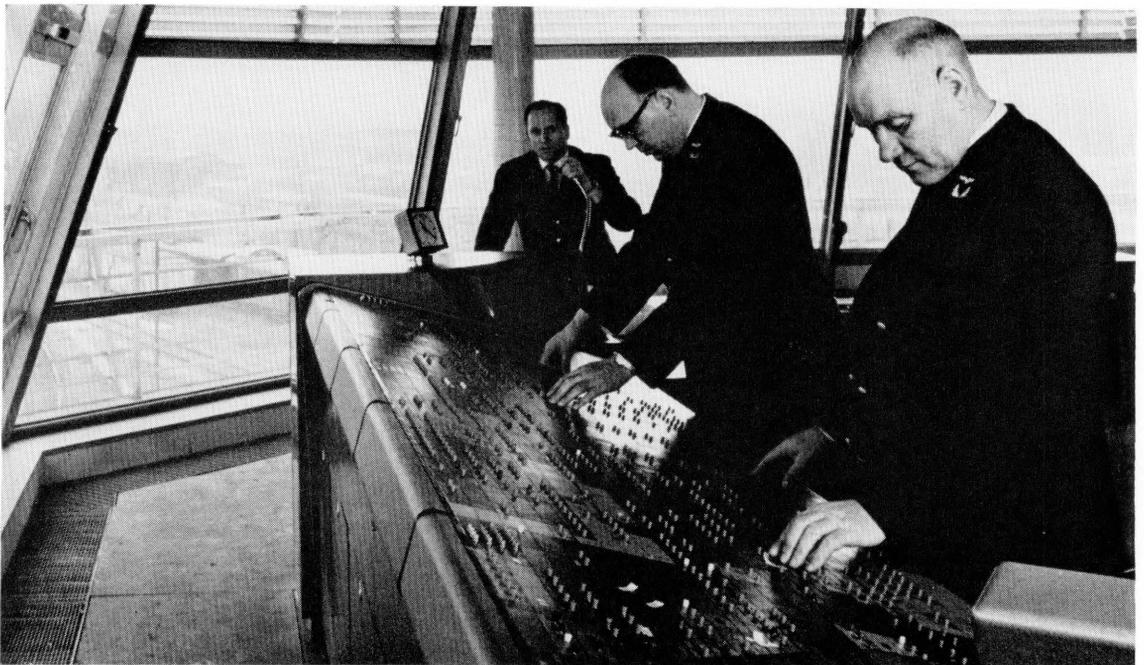
Figure 5—Operating desk at Oldenburg, Germany, of track-diagram railroad switching installation.
