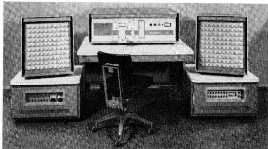
Figure 7—Console flanked by two 100-circuit indicator panels of the Digitor 400 multiplex alarm monitoring and recording system.
